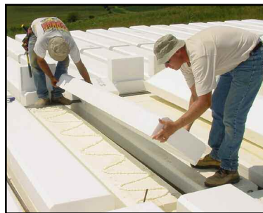
Foam glue is used to attach top-hats to the base section.
