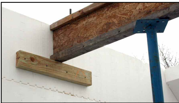
Shoring beams are supported against adjoining walls with dimensional lumber.
