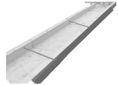
Frost Protected forms are placed on level ground backfilling sides with gravel and/or dirt approximately half the height so forms stay in place when poured
