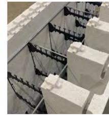
Many installers will place In-Wall bracing at the course of brickledge blocks. This will help in keeping wall alignment and enforcing the brickledge.
