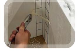
Add the 3rd zip tie to the inside of the corner and pull it tight. **IMPORTANT - Remove zip ties after concrete is set.**
