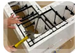
Place a LiteForm ICF 90° Corner Tie onto the pre-molded slots. You may need to clean the slots with a drywall saw. Tap the corner with a hammer so it is flush to the
