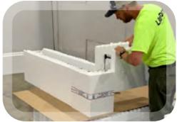
Repeat the same steps from the 1st course using the other 1/2 block on the alternate side of the LiteForm ICF 90° Compact Corner. This will create an alternating seam for your wall.
