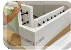
Slide both the full and half blocks onto the compact corner.
