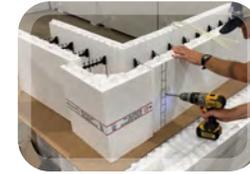
Drill or punch a hole on the opposite side of the 1st plastic tie on **both** sides of the 48" adjoining block.
