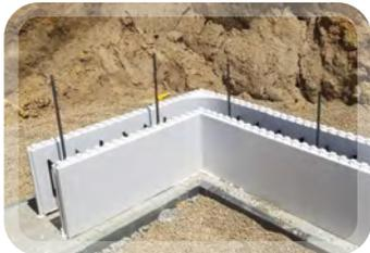
Using low expansion foam adhesive, run a bead of glue along the bottom side of the LiteForm ICF 90° Corner Block. Set the Corner Block in place on the footing following the chalk line. Glue will normally set within 20 minutes.
