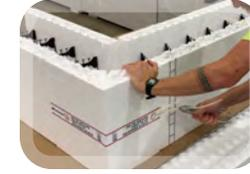
Using the provided zip ties, run ties through the pre-drilled holes in the corner and into to the hole you made in the adjoining block. Pull the zip tie tight against the ties.
