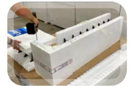
Drill or punch a hole on the opposite side of the 1st plastic tie on both sides of the 24" cut block.
