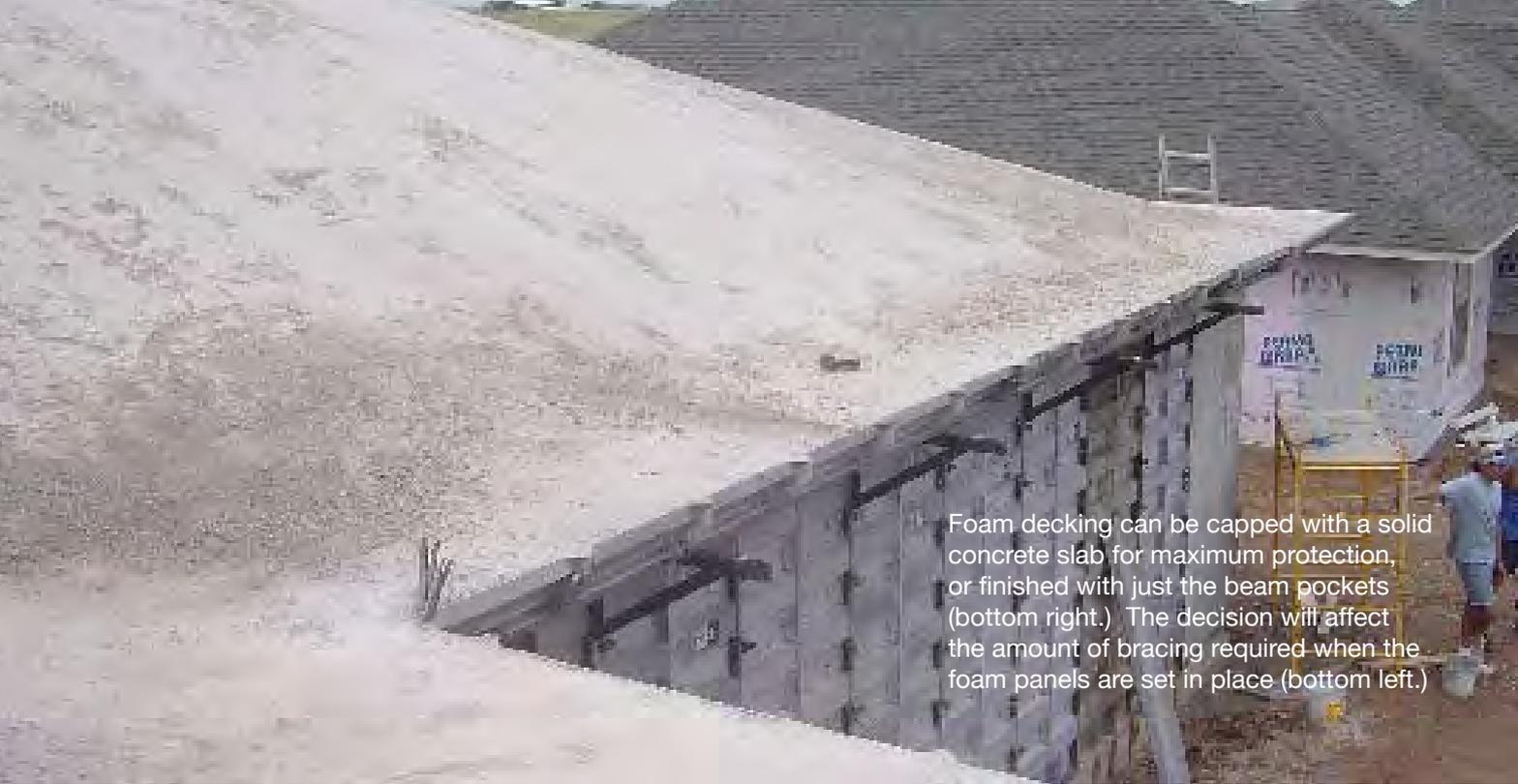
Foam decking can be capped with a solid concrete slab for maximum protection, or finished with just the beam pockets (bottom right.) The decision will affect the amount of bracing required when the foam panels are set in place (bottom left.)
