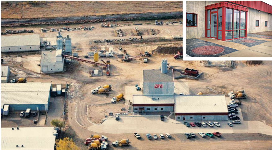
This aerial view of the Dickinson Ready Mix Co. property, shows the new plant (center) and the old plant (upper left), which the company was only going to use as back-up, but unusually high demand kept it open for the duration of 2011. The plant's front entrance (inset) features decorative concrete work, including exposed aggregate concrete, as well as stamped and imprinted concrete.
