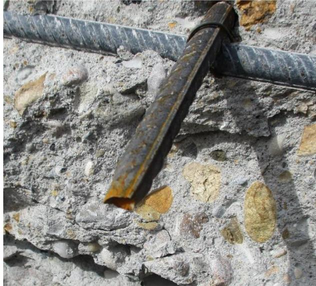
Figure 8: Rupture of Steel bars
