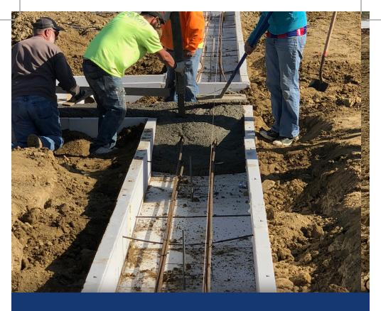
3. Rebar is placed to reinforce LiteFoot for added strength and support.
