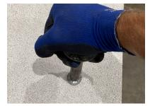
Place push washers onto pins using a aligning the pins to the pre-drilled holes. push pin tool or 5/8" deep well socket.
